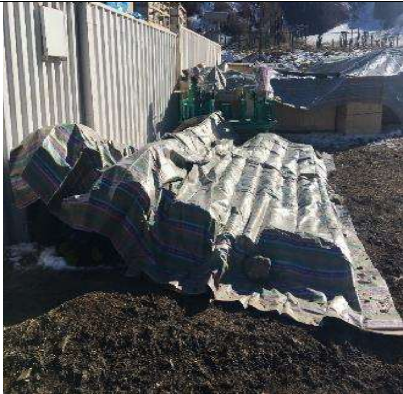
Material and equipment storage at Kobi Site for Lot#1
