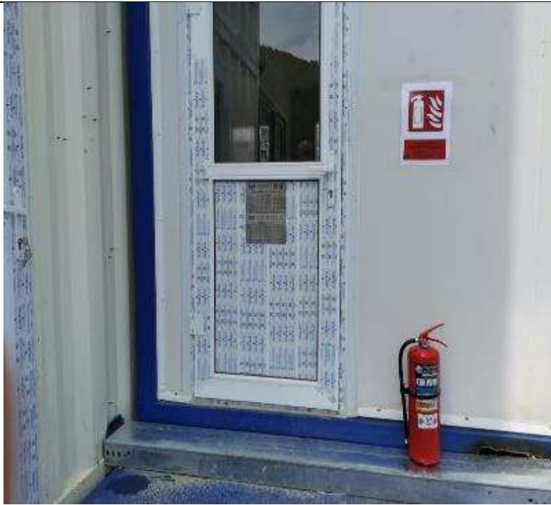
Fire Fighting arrangement at Kobi Site Lot#1
