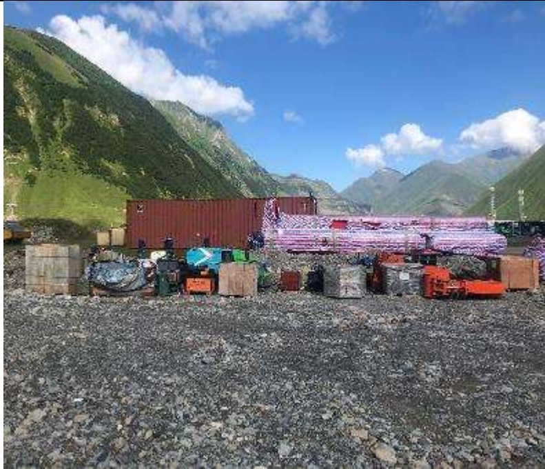
Material storage at Kobi Campsite
