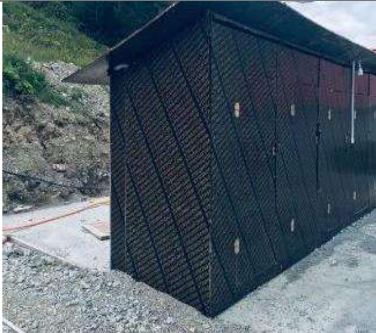
Temporary arrangement of toilets at Kobi site
